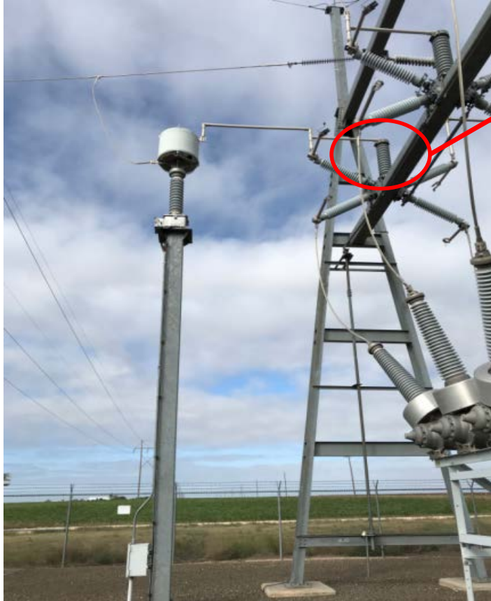
Lightning arrester
